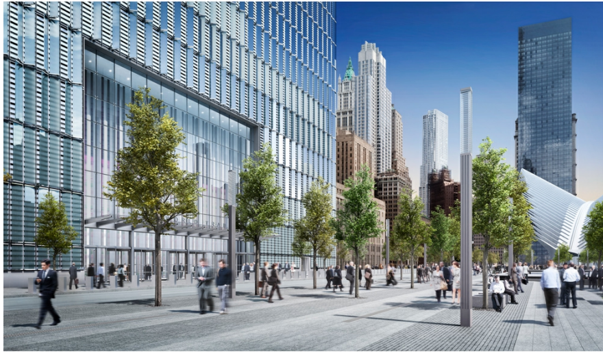
Overview of a street-level entrance of One World Trade Center. Image: PANYNJ/ Durst Organization
